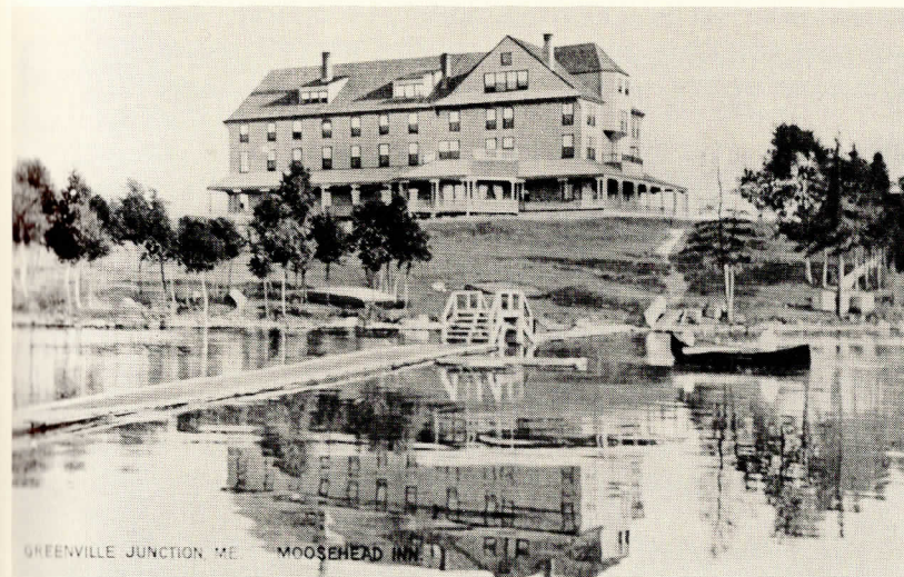
The Moosehead Inn, Greenville Junction.
